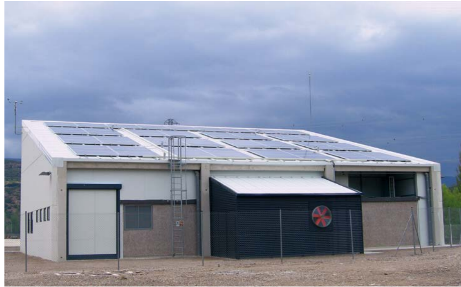
Parte trasera Microrred. Rear of Microgrid.
