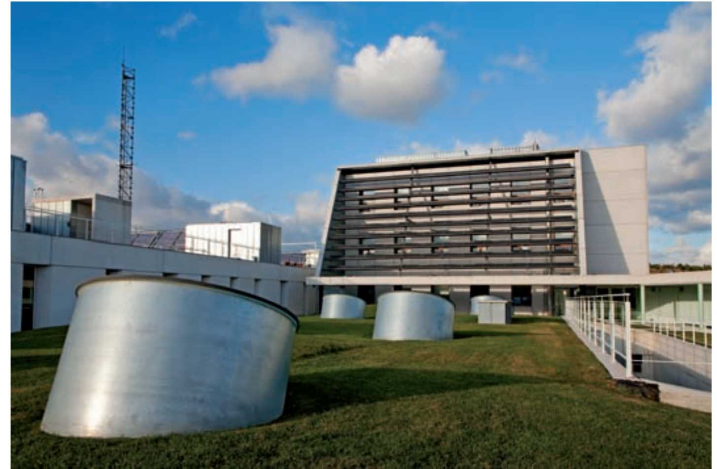
▲ Edificio CENER. CENER building.
