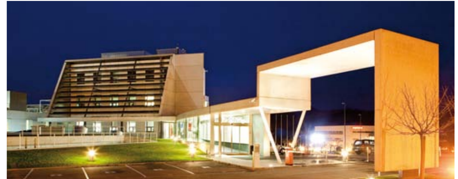
▲ Edificio CENER. CENER building.
