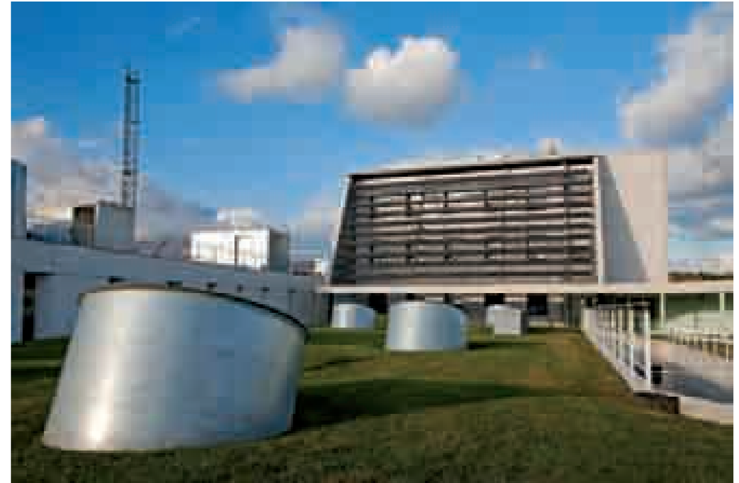
▲ Edificio CENER. CENER building.
